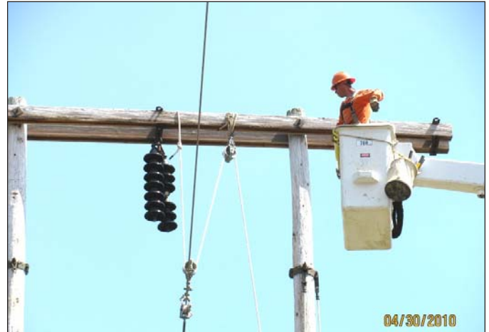
A6 Jeremy Harris lowering conductors on highline job in Ithaca, NY for Harlan Electric
