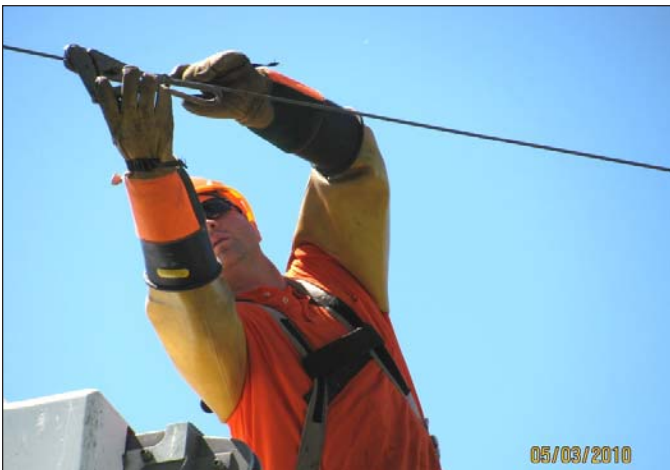
JL Tim Pearce, Harlan Electric Distribution Job, Fulton, NY - May 2010
