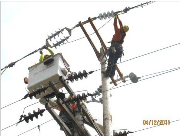
1249 JL Richard Hack's Crew Harlan Electric, Sub T - Saratoga, NY
